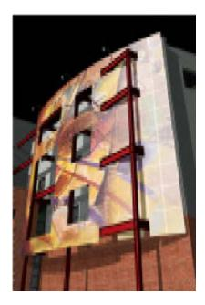
The designers selected a raw exterior character of metal siding above first-floor brick laid in irregular forms. To complete this "loose fit" enclosure that welcomes clients and meets the low budget, the red structural frame is pulled outside.
