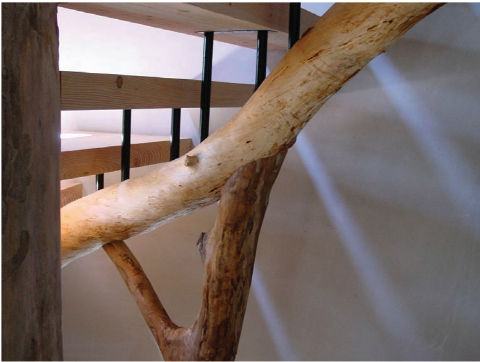
An open stairwell was crafted from pieces of beech saved from an in-fill project in Portland and spruce branches from a tree on the property. Photo courtesy of the Oregon Department of Energy.
